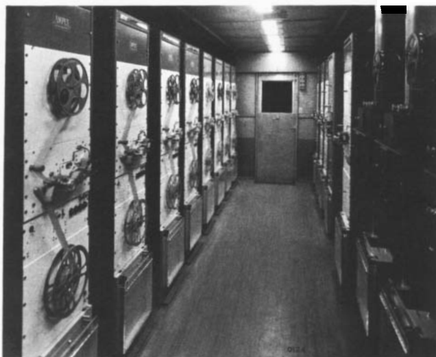
Magnetic film transports are used extensively in the motion picture industry for dubbing master sound tracks. Here is the Ampex 35-mil film transport installation at Glen Glenn Sound Studios, Hollywood.
