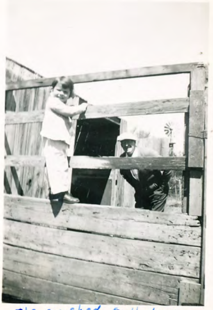
The cowshed fell down and Grandpa rebuilt it
