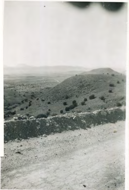
HWY 118 BIG HILL before being paved.
