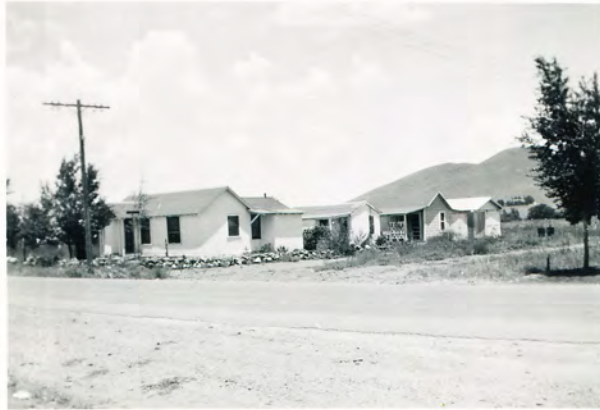
HWY 118 ONE LANE WID E. NATIONS UNPAVED
