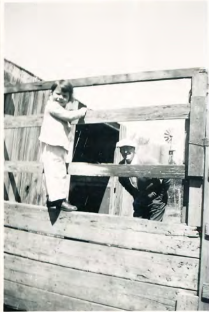
1948 The cow shed fell DOWN - GRANDPA FIXED IT
