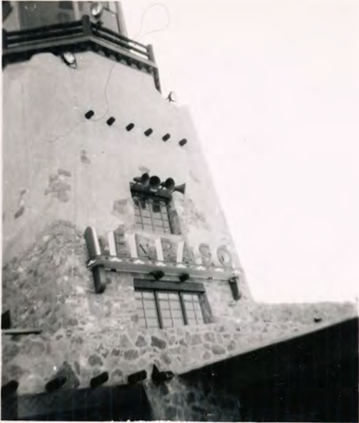
Fort Bliss / El Paso Airport 1951
