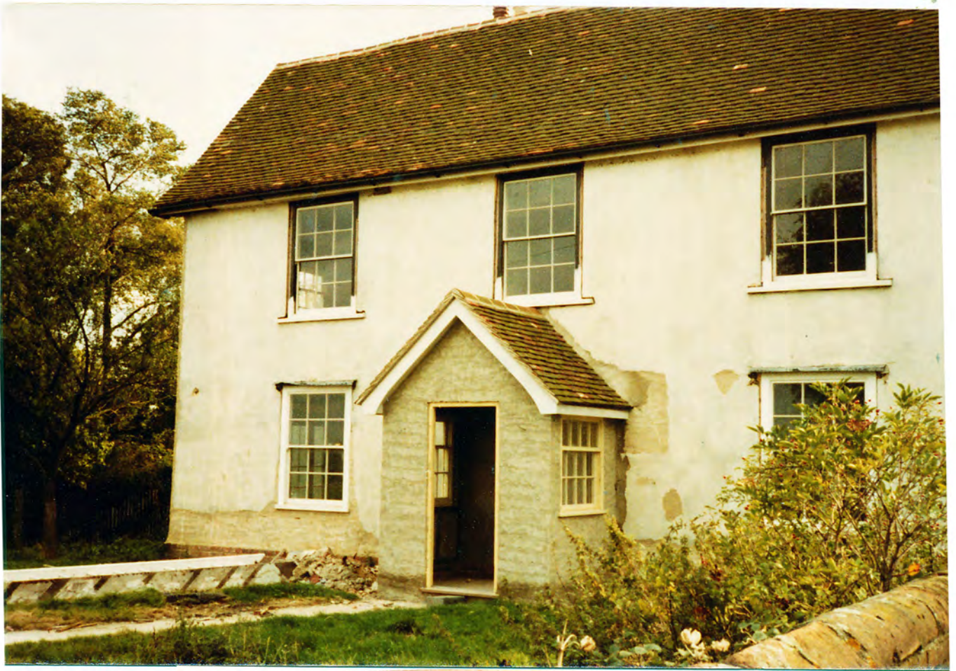
Cuckoo Eye Farm in process of being renovated Nov 1980
